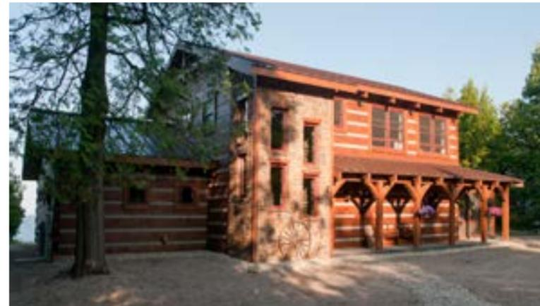
Stone is a beautiful complement to wood. The stairwell tower was faced with a mix of stone. For the exterior, real 6-inch veneer stone was used. On the interior, manufactured stone was used due to space and weight-bearing constraints. The tower also features a back-to-nature rustic staircase that incorporates tree trunks and twigs.
